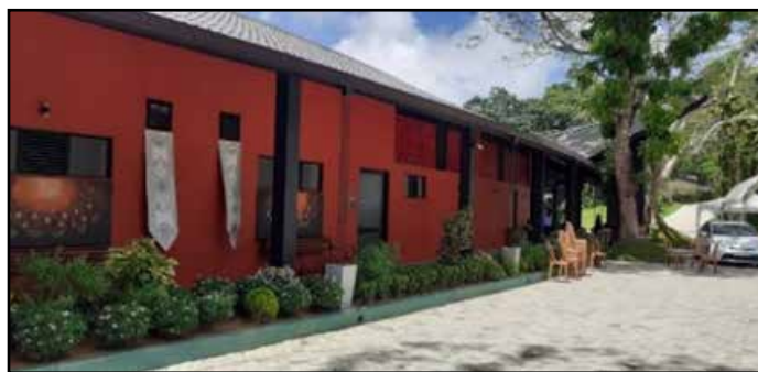
With the aim of strengthening functions of Palliative Care Consult Services in cancer treatment hospitals, NCCP provided funds to Palliative Care Units at TH Karapitiya and BH Thelippalei to procure necessary equipment
